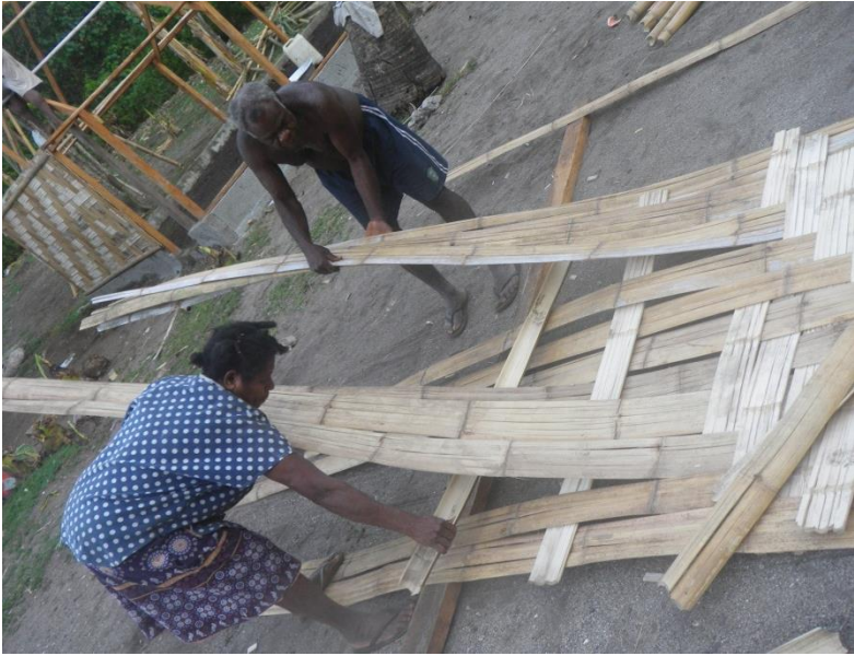
Figure 5: Vet 'weaving' flattened buvat 'strong bamboo' into a wall panel
