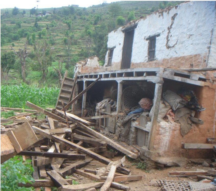
Figure 4. After the 2015 earthquakes. Image © Ningmar Syuba.
